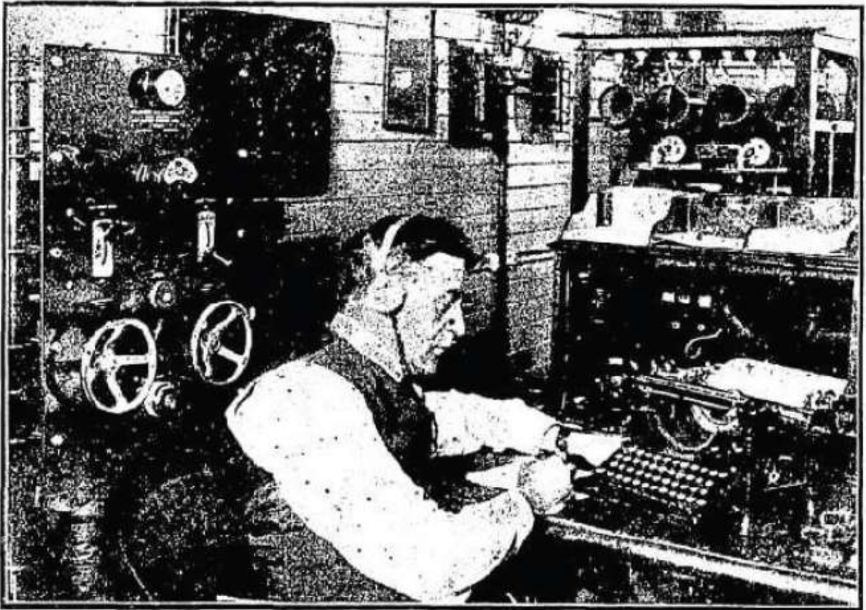
The interior of Hobart Commercial Radio Station, showing the new apparatus installed recently. The control panel may be seen at the left of the picture and the receiving set in front of the operator.
